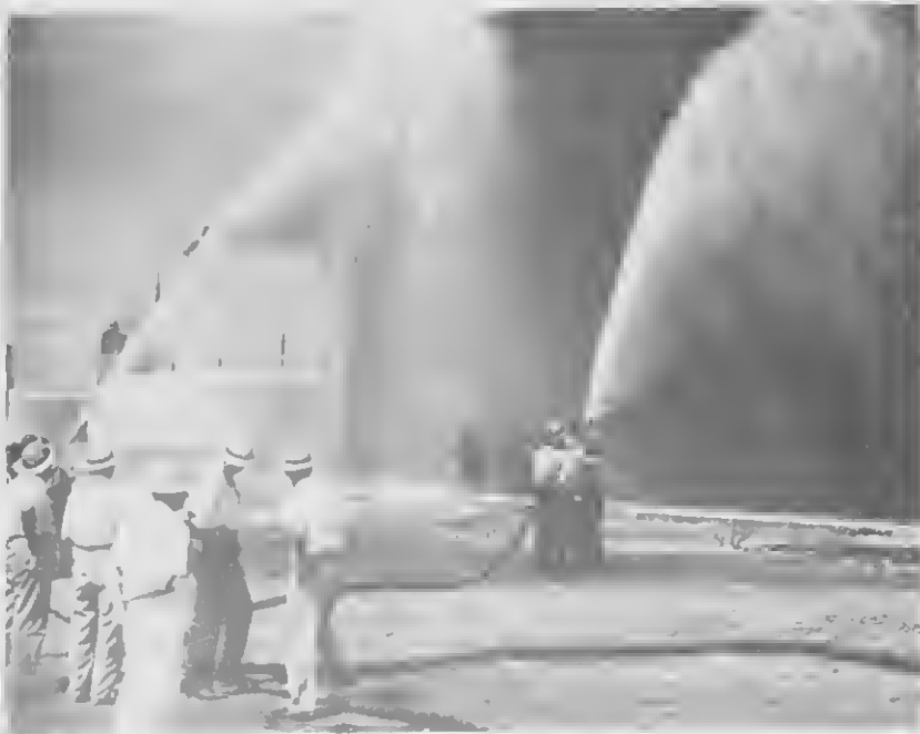
DURING One of Lago's regular fire drills, shell plates of a tank are cooled down by fog.
